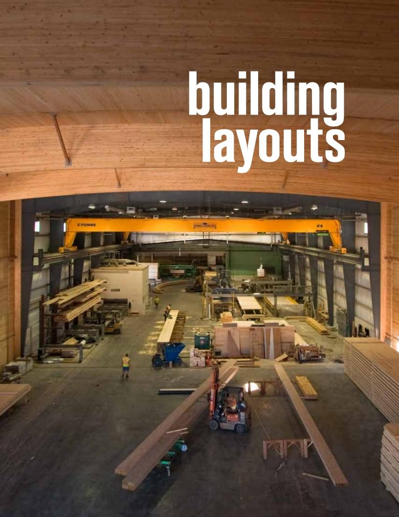
There are two basic types of industrial buildings: open span with open interior space and structural supports at the perimeter of the building, and multi span buildings with interior columns. Deciding which of these layouts should be used depends on the requirements of the production process. Some processes require long spans and full flexibility of the interior layout, and others can easily accommodate one or two rows of internal structural supports.
