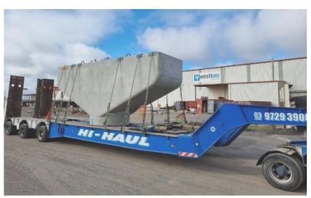
Complete precast bridge crosshead delivery to site [Credit Westkon Precast]
