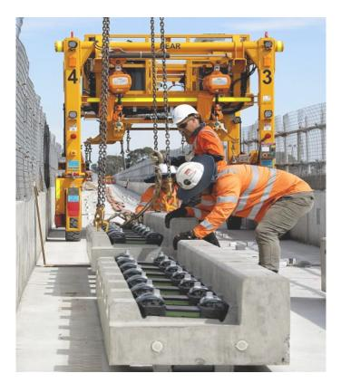
Specialist designed lifting system for handling prefabricated rail precast components [Credit LXRP]
