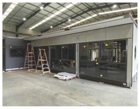
Final inspection on completed module [Credit ATCO]
