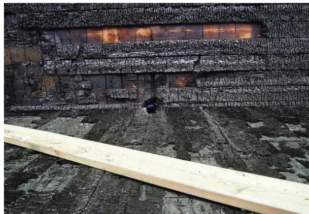
(d) zoom into the junction (underside)
