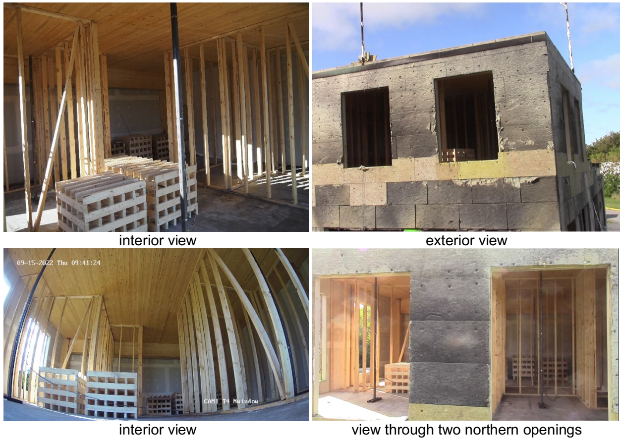
Figure 49. Under-construction suite for Test 4 (before testing).
