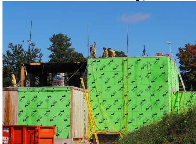
removal of roof cover to attack outside
