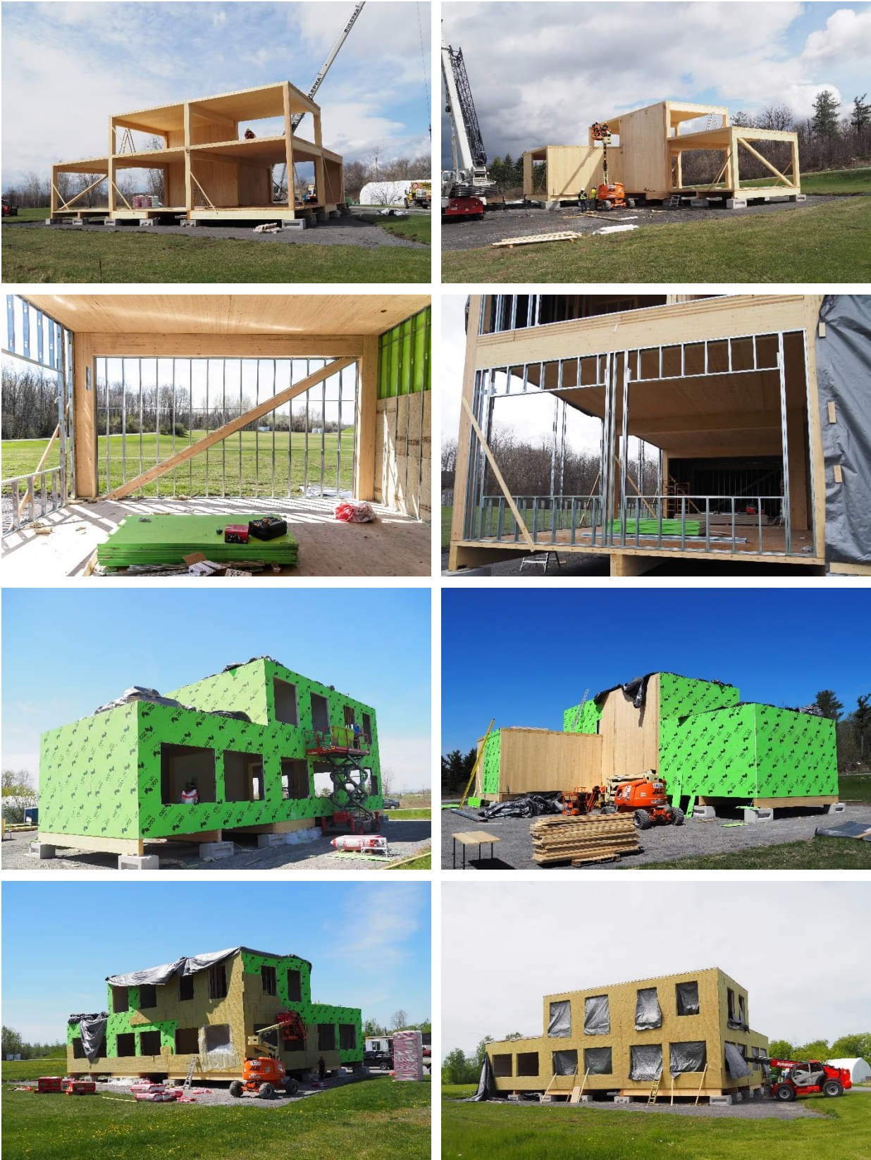
Figure 3. Photographs of mass timber test structure during construction.
