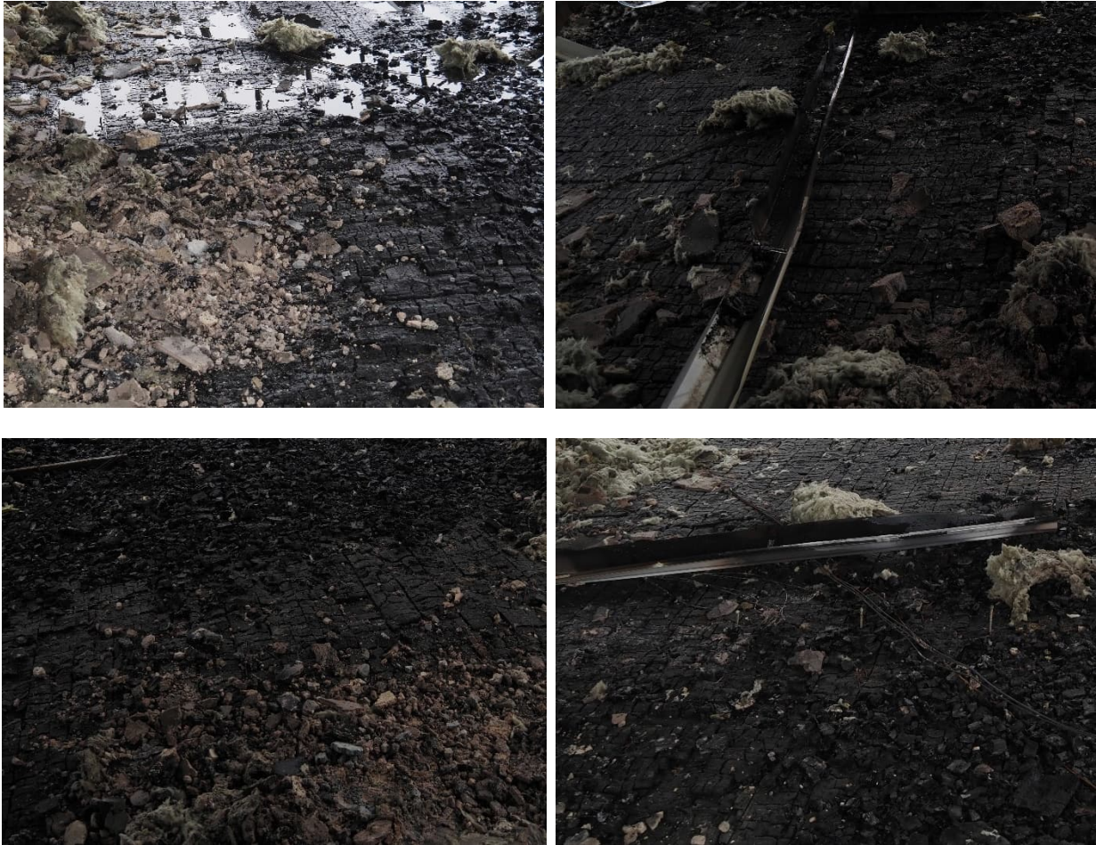
Figure 56. Charring on CLT floor (Test 4).
