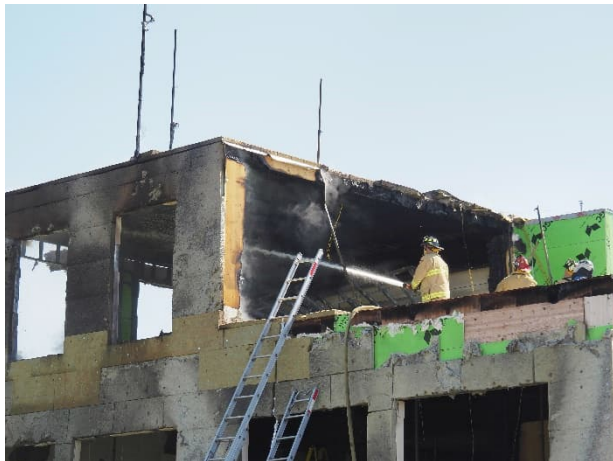
removal of exterior walls to attack outside
